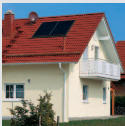
Afb. 16: Vlakke collector Vitosol 100, type 5DI
